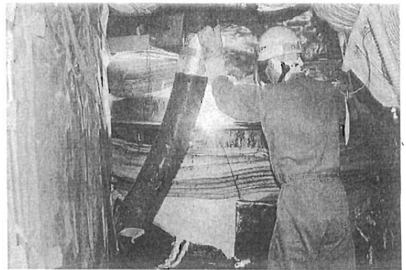
Photo 3 Electric welding of cylinder bottom to reactor pressure vessel
